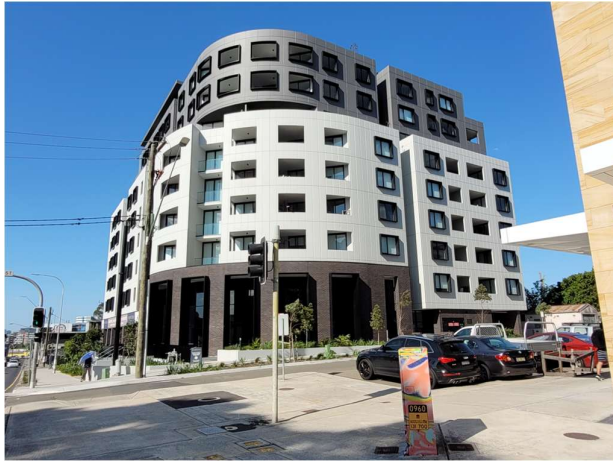
Figure 3 – Photograph of 96-102 Princes Highway Arnccliffe viewed from the Princes Highway
